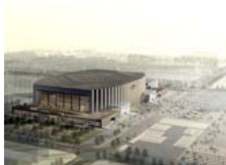
Beijing Science and Technology Gymnasium
