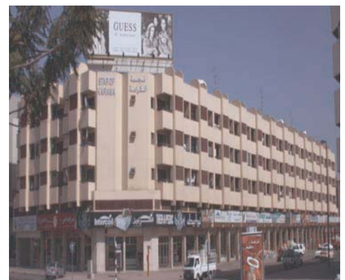
Karama Building - UAE
