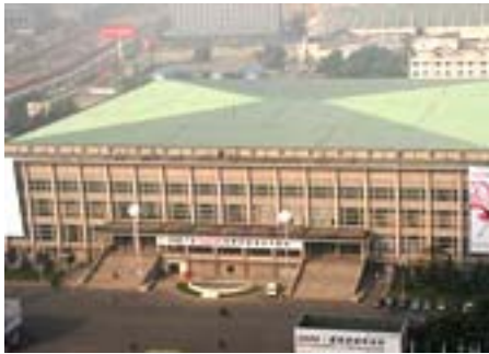
Capital Indoor Stadium
