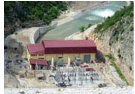
Kejiah Power Station - Macedonia
