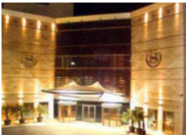
Sheraton Hotel - KSA
